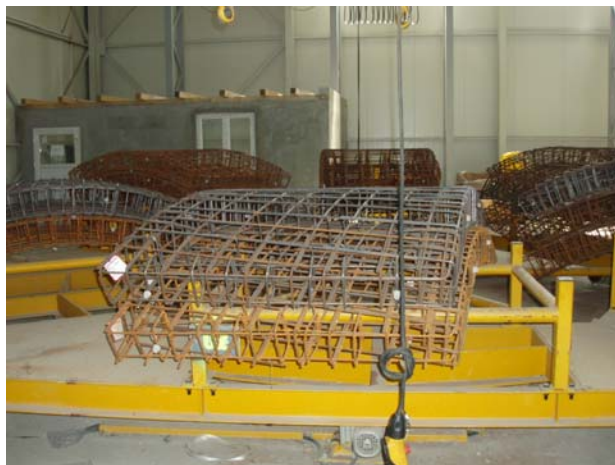
Photo3-4. Assembling iron reinforcing bar for segments of Interceptor
